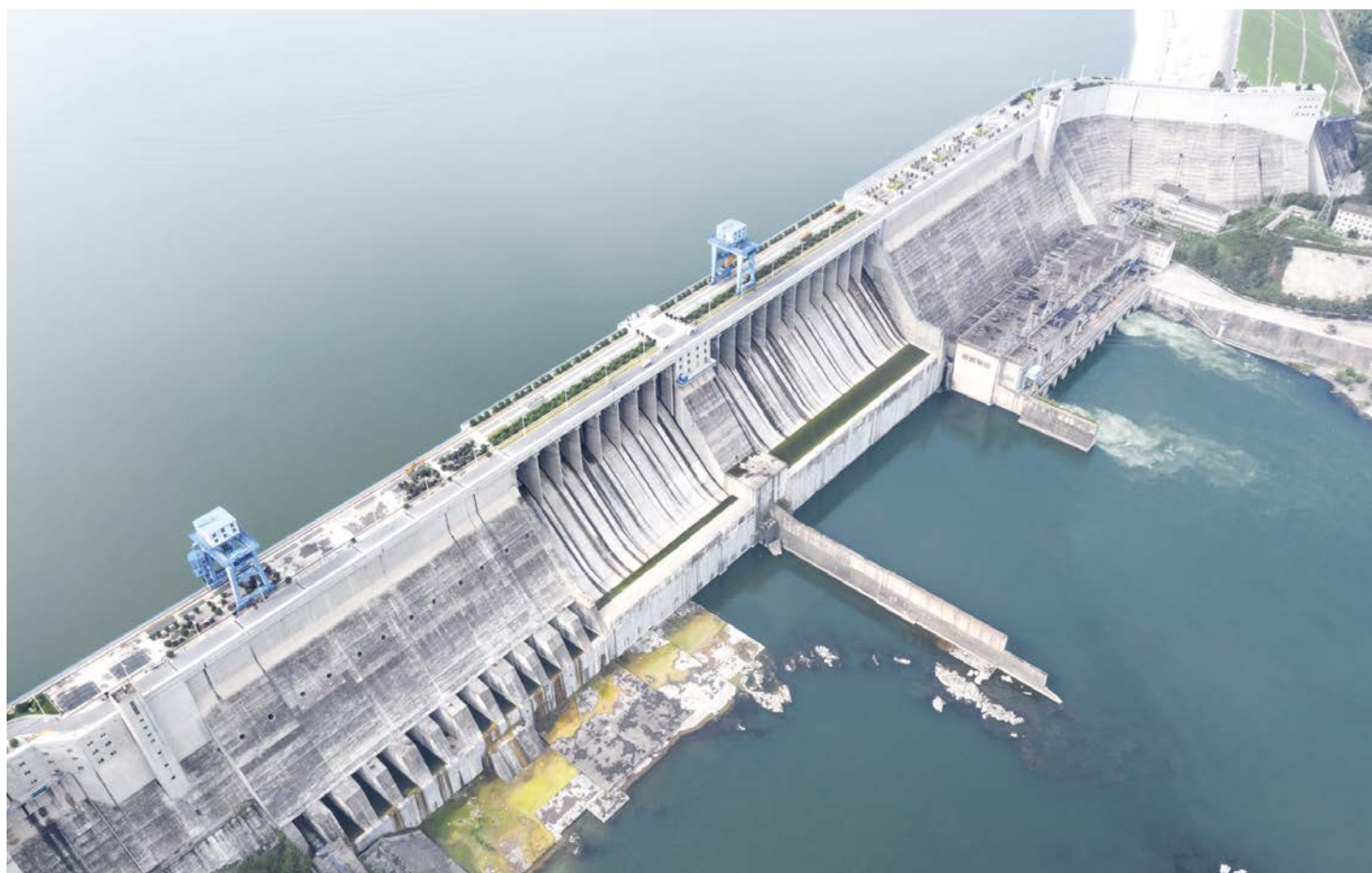
Hydroelectric dam on Danjiangkou reservoir, China | Gettyimages
