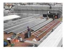
In 2011, a photovoltaic plant (PV) was installed on the roof of the Flur Süd building in Zurich. The system consists of 360 high-performing solar modules with a capacity of 90 kWp, allowing UBS to generate 83,000 kWh of solar power each year, equivalent to the annual consumption of 20 Swiss households. 16 UBS employees volunteered to help set up the PV, thus gaining valuable insights on how a PV plant works and is installed.
