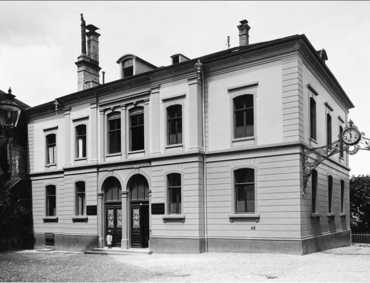
The branch of Union Bank of Switzerland in Lichtensteig, 1914
