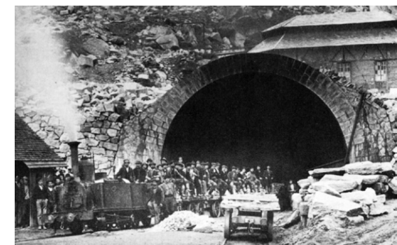
Construction of the Gotthard tunnel, 1880
