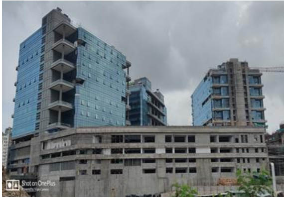
Building 5 – Podium level RCC work in progress
