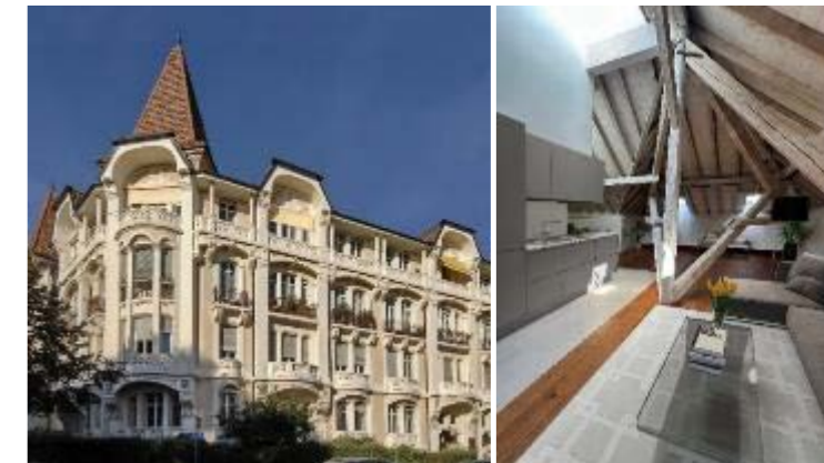
Lausanne, SAED-SIMB | Residential buildings Attic conversion
