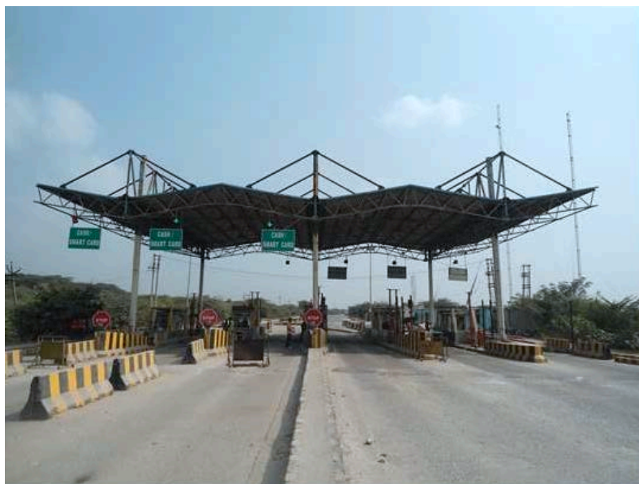
Figure 1:1 Toll Plaza on Crusher Zone Road
