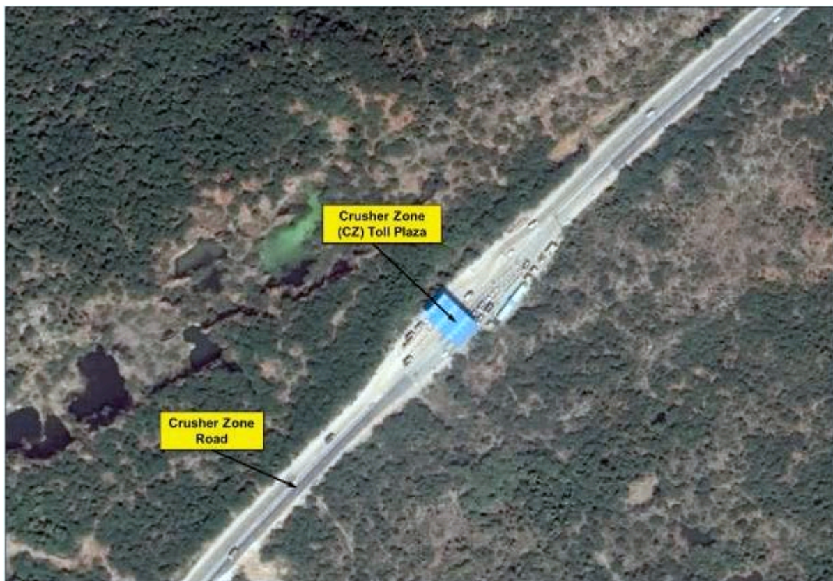
Figure 1:6 Existing Toll Plaza Location near Crusher Zone on Crusher Zone Road
